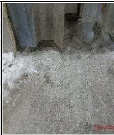
Ice formed on floor at entrance of cold storage, the floor is slippery, Cold storage needs proper stacking of m/c.
