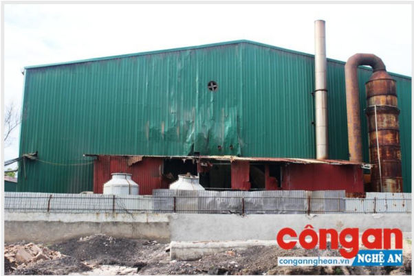
Scene outside where the boiler explosion occurred
