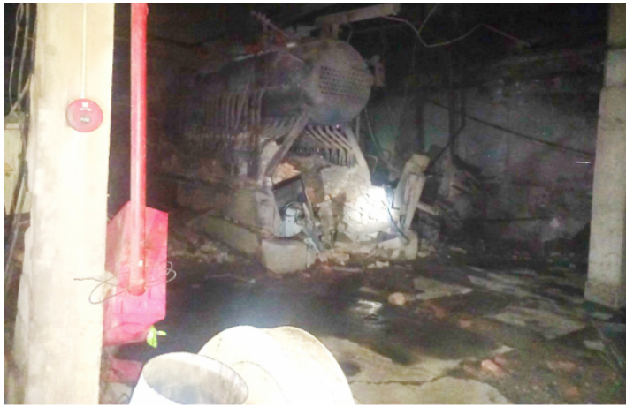
Close-up of the explosion scene.
