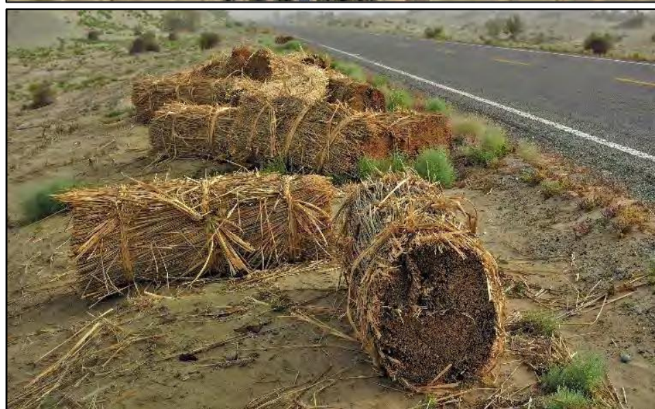
Tarim Desert Highway protected by 'Green Wall', Reed straw delivered to the roadside for safety work
