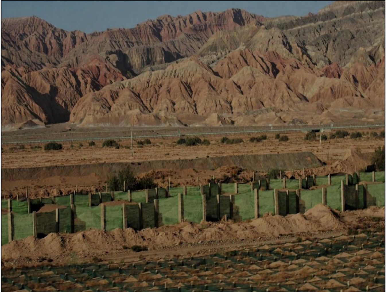
Windbreak on the G 314 and the parallel Kashgar-Aksu railway line 1
