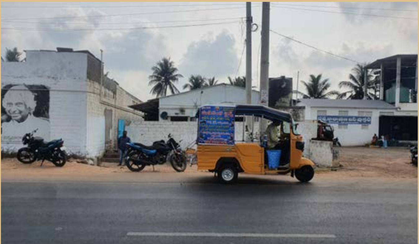
Peeling sheds in Tallarevu (Andhra Pradesh, 2022)
