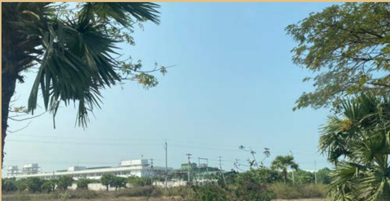
A large shrimp processing facility (Andhra Pradesh, 2024)
