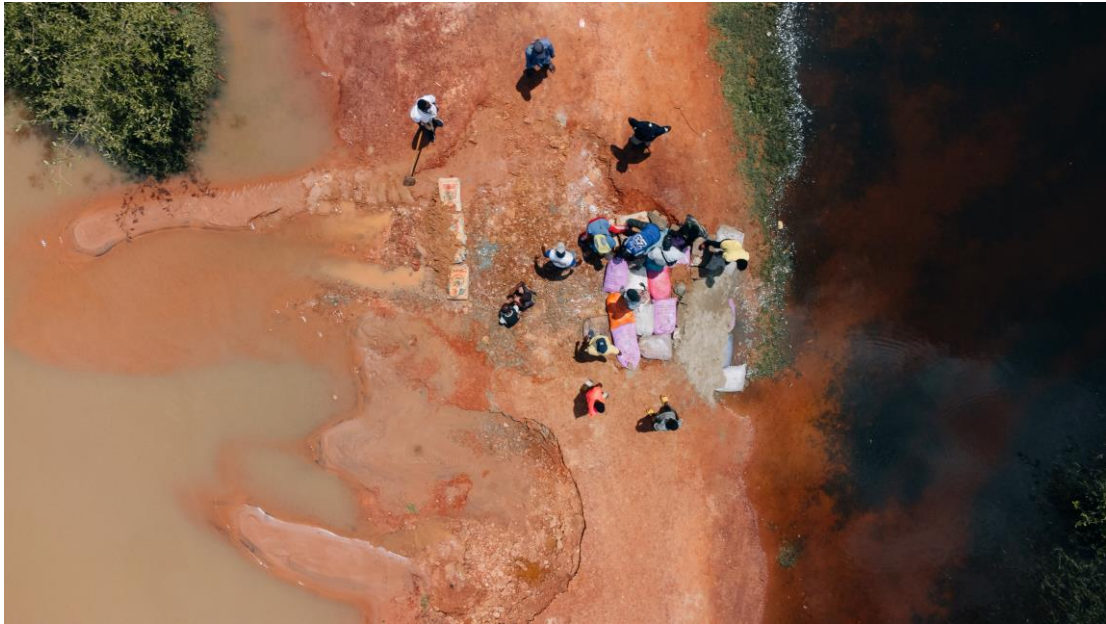
↑ Sanyang residents attempting to repair the broken road ©Julian Hahne/Amnesty International
