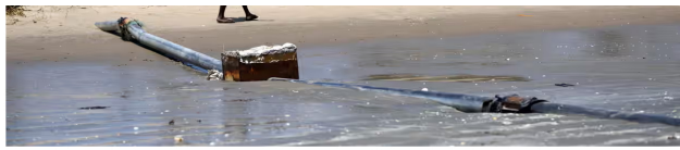
A waste pipe belonging to Golden Lead
