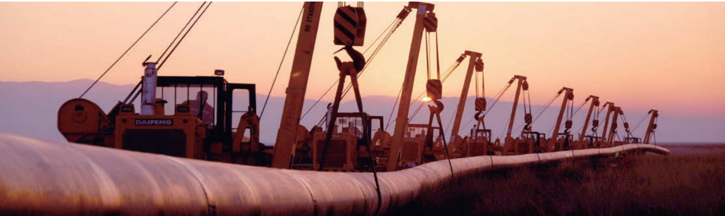
↑ Pipeline laying site
